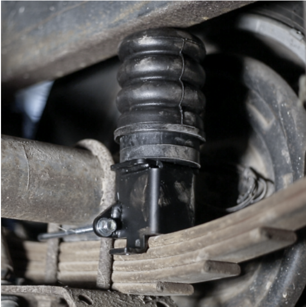
TRAILER SUMOSPRING INSTALLED
